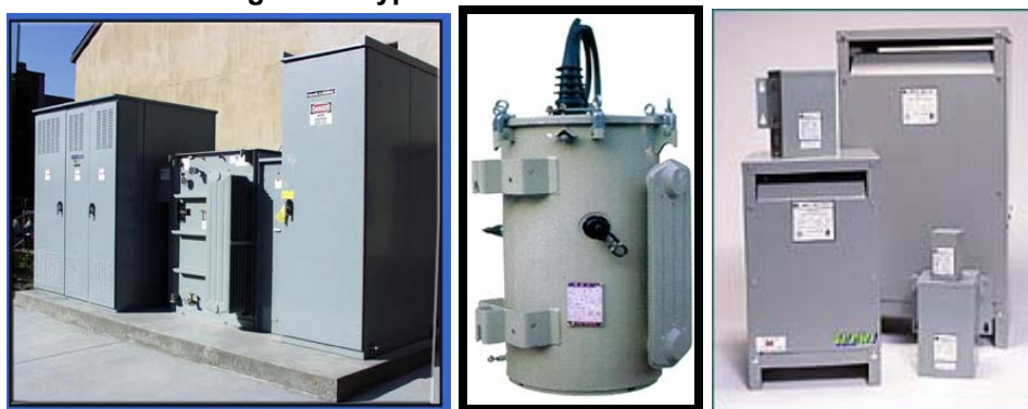
Figure 6. Typical Distribution Transformers
